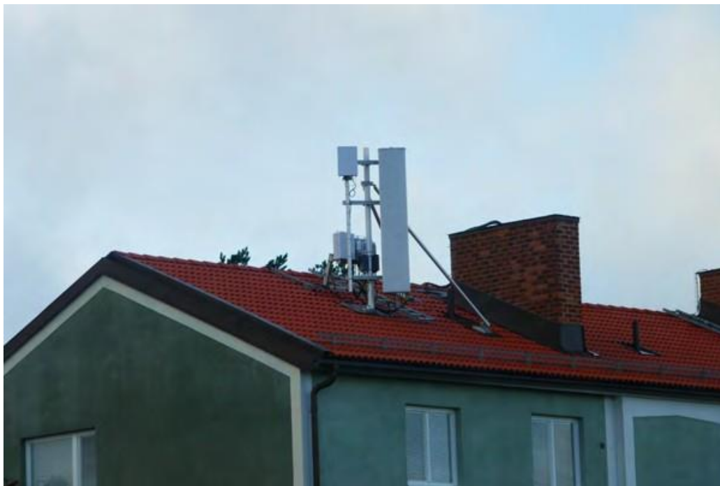
Figure2: 5G base station on the roof of a three-floor building located 60 meters from the study apartment
