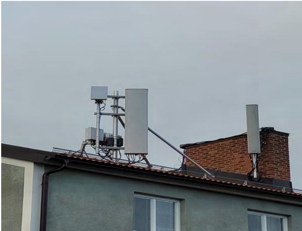
Figure 3: 5G base station on the roof of a three-floor building located 60 meters from the study apartment. Initial figure after the 5G installation showing the previous base station attached to the chimney
